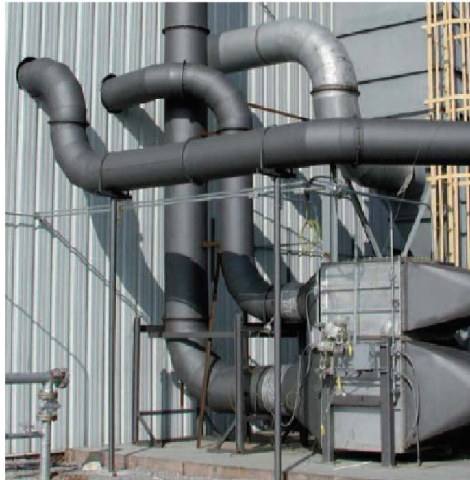
Energy recovered from an aluminium furnace exhaust being used to pre-heat the incoming air to the furnace
