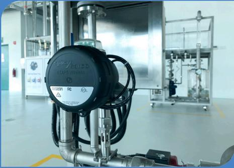
It provides a clear indication on steam trap performance and enables steam system operators to determine when and where to deploy trap maintenance so that budgets can be controlled. With user-defined reporting functions, the system can be set or adjusted to generate updates as frequently as required.
