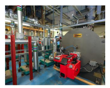
In order to get the system back to its optimum operating level, Spirax Sarco replaced a number of traps and valves, and provided a valve refurbishment and reconditioning service to extend the life of some of the worn components.
