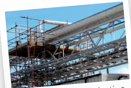
Steam diversion & eliminating oversize main
