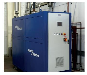
generator 50 kW (50 kg/h @ 3 bar) with preheating capability and the ability to control feedwater quality.
