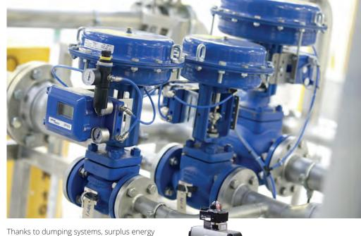
Thanks to dumping systems, surplus energy in the ships steam network, can be recovered, stored and re-used by introducing a Hot Well (at temp. 95 °C).
