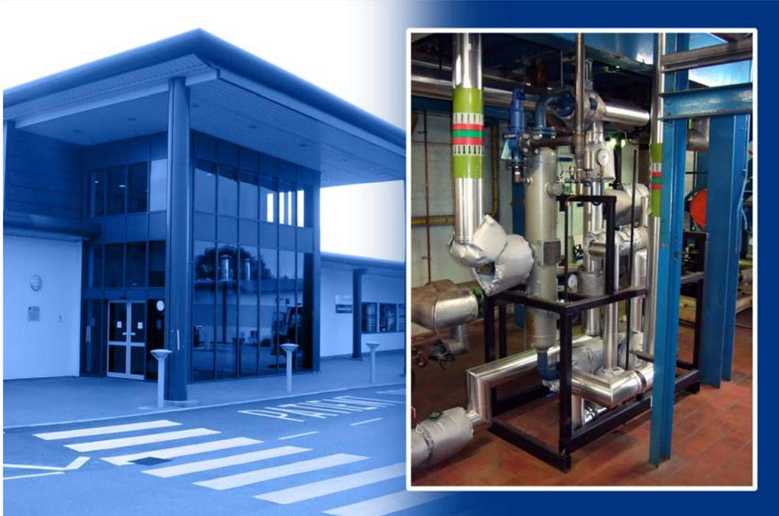
*Leighton Hospital improved energy recovery and has reduced its carbon emissions by around 95 tonnes a year, cutting fuel bills by more than £10,000.*
