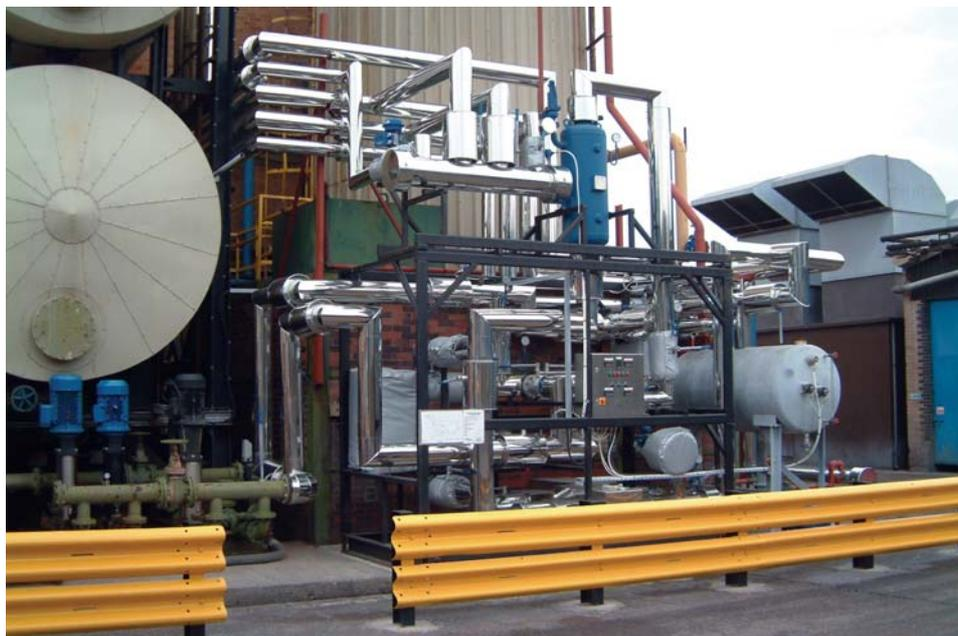
*A Spirax Sarco flash steam recovery system is delivering direct energy savings of 10% plus a further 10% in indirect savings at De Mulder & Son.*
