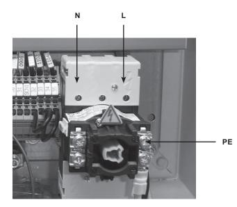
Fig. 7 Version with single-phase power supply
