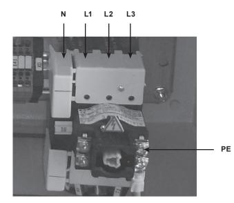
Fig. 8 Version with three-phase + N power supply
